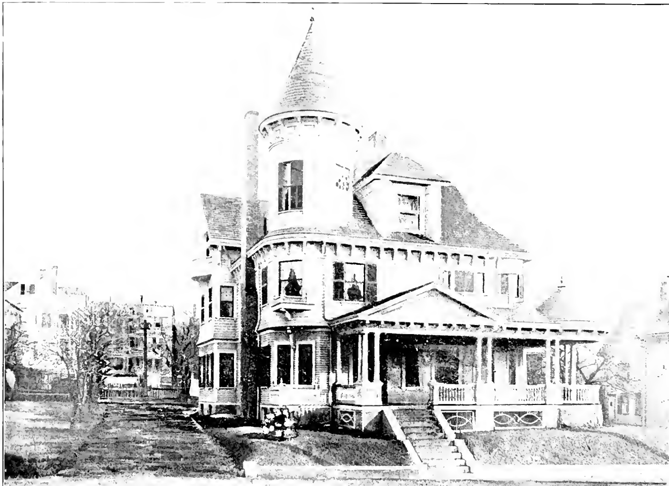
RESIDENCE OF DAVID M. DILLON, MYRTLE AVENUE.
