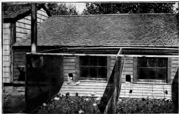
View of Part of Exterior of Brooder House
