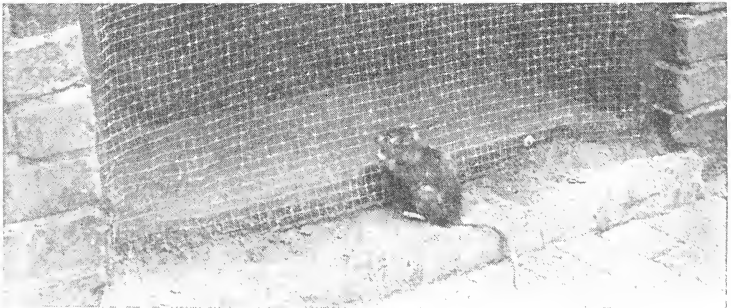
Figure 12.—Hardware cloth is useful in excluding rats from openings that cannot be closed with brick or mortar.
