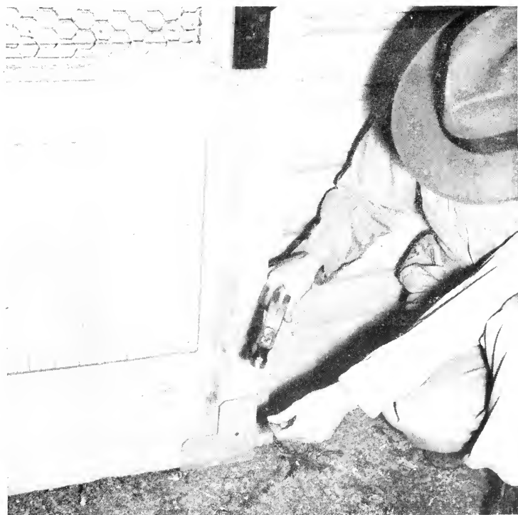
Figure 13.—Edges of doors or other openings where rats gnaw should be protected with metal sheathing.
