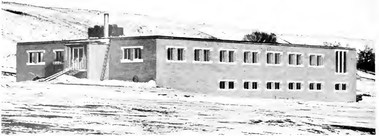
The Jamestown administration building and laboratory, headquarters of the new Northern Prairie Wildlife Research Center established to serve the "pothole" country of Minnesota and the Dakotas, the most important waterfowl breeding ground in the United States. (Photo by Harvey K. Nelson)
