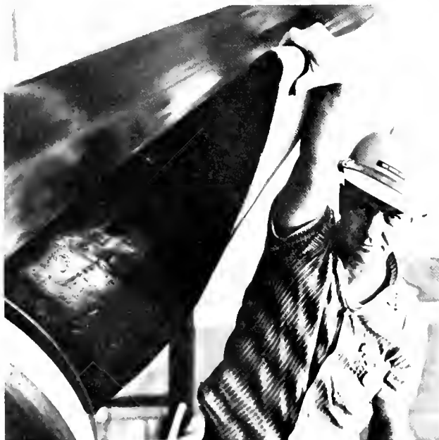
FIGURE 36.—Blade of Kaplan turbine at Bonneville Dam. The blade has thick edges, but fish are injured where the clearance between the turbine blade and the turbine wall is minimal.
