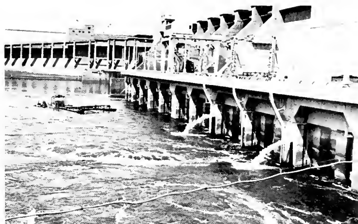
FIGURE 37.—Fish released into turbines at Iee Harbor Dam were collected below the dam. Comparisons were made of the survivals of fish that had passed through turbines and fish that had bypassed the turbines. The hose in the foreground carried the fish that were bypassed.
