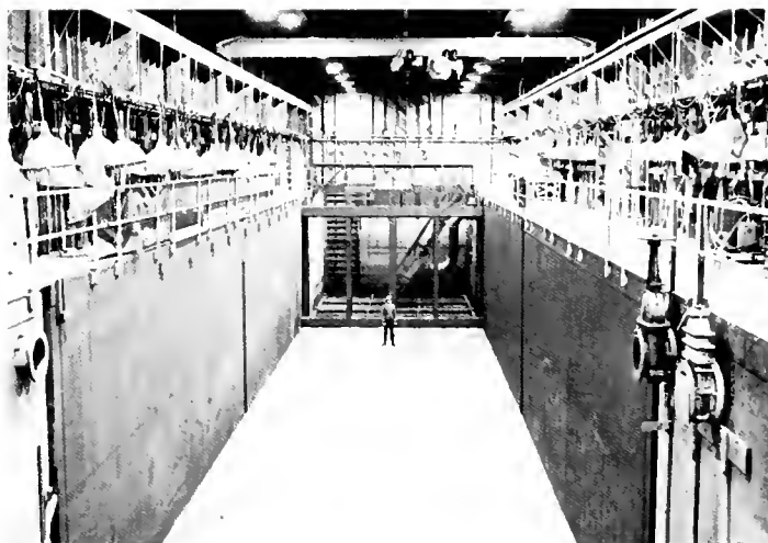
FIGURE 24.—TOP. The Fisheries-Engineering Research Laboratory (arrow) at Bonneville Dam on the Columbia River. BOTTOM. Drained test channel inside laboratory.
