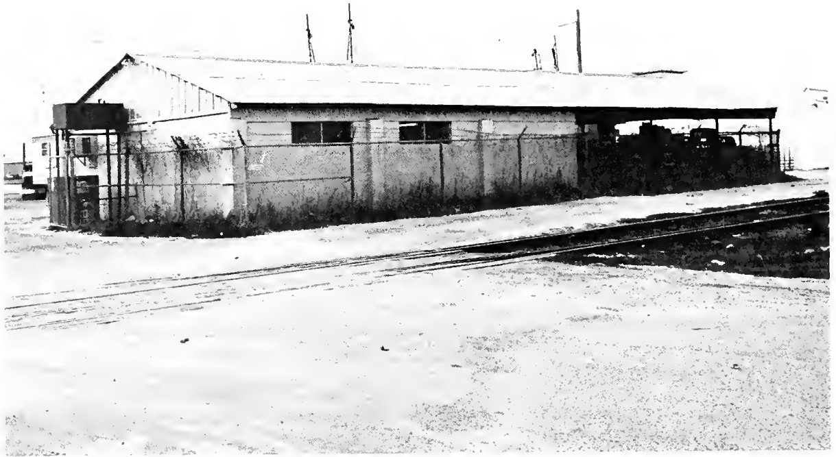
Figure 1.—Concrete block structure housing the seawater recirculation system and laboratory at the Exploratory Fishing and Gear Research Base's dock site on the Pascagoula River. One of the elevated filter boxes can be seen at the end of the building. The saltwater well is located beneath the filter box.
