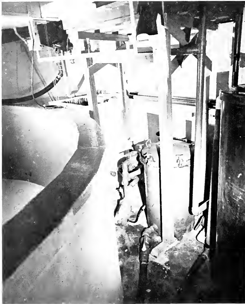
Figure 6.—A portion of the recirculation system occupying the south wall of the laboratory. The experimental pool, sump, pump, diatomaceous-earth filter, and 500-gal fiber glass tank are shown from left to right.
