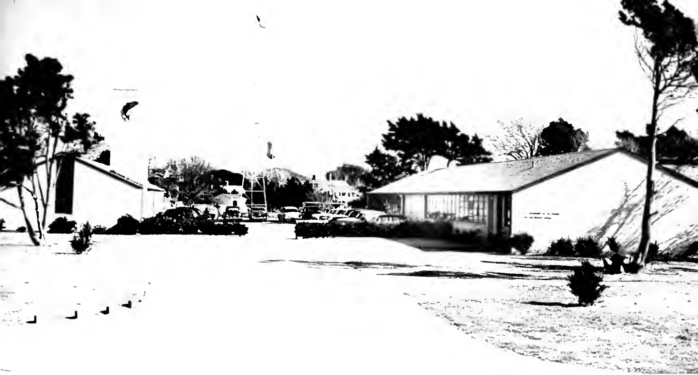
The fishery laboratory, service maintenance building, new concrete driveway and parking area. The maintenance building (on the left) houses the garage, shops, and pumping and heating facilities, and provides storage space
