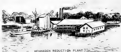
MENHADEN REDUCTION PLANT
