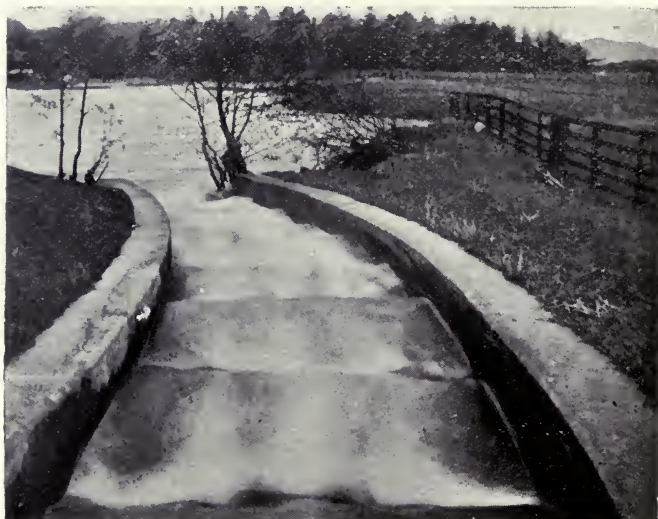
BOTTOM OF FISH-PASS AT DUPPLIN DYKE.
