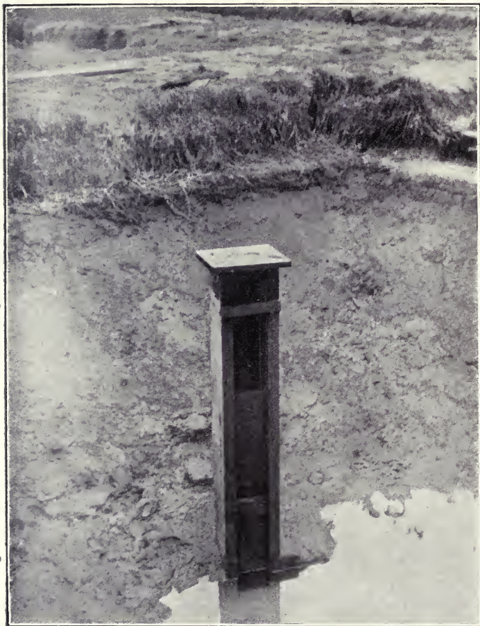
A CONTROLLING SLUICE FIXED IN AN EMPTY POND.
