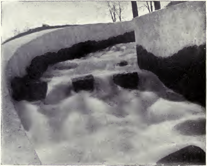
A FISH-PASS, SHOWING ARRANGEMENT OF BOULDERS.
