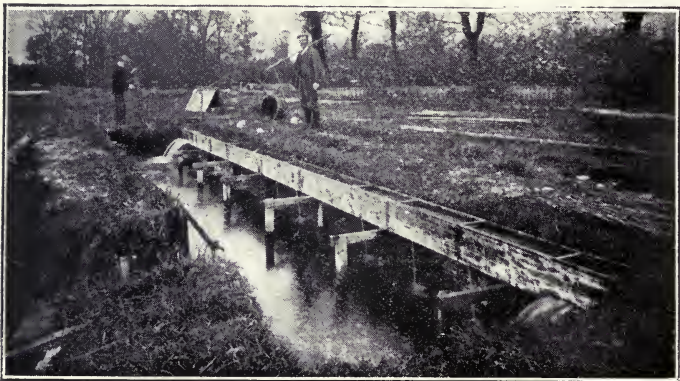
AN OVERHEAD HORIZONTAL BOX SCREEN.
