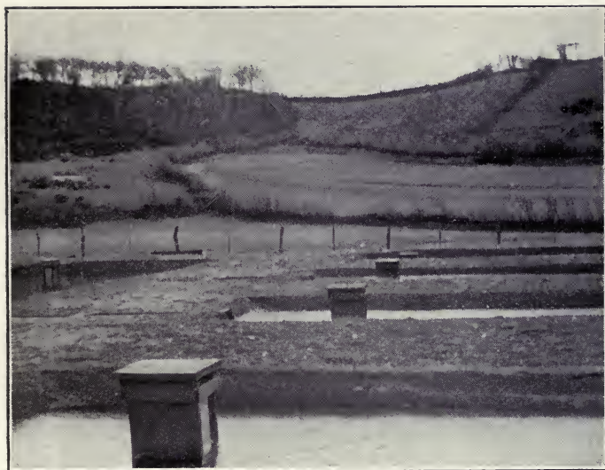
CONTROLLING SLUICES IN PONDS.
