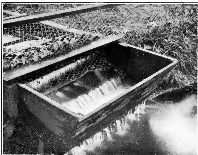
CONTRIVANCE FOR PREVENTING FISH RUNNING UP SURPLUS WATER CHANNELS, ETC.
