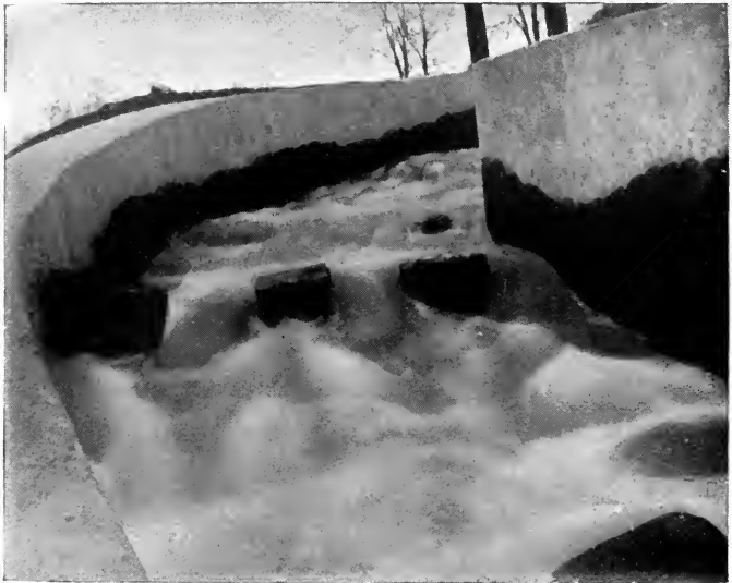
A FISH-PASS, SHOWING ARRANGEMENT OF BOULDERS.
