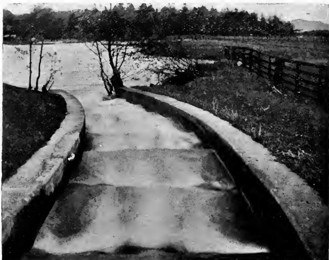
BOTTOM OF FISH-PASS AT DUPPLIN DYKE.
