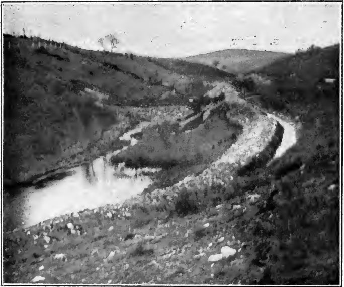
DAM AND SURPLUS WATER CHANNEL IN THE HILLS.
