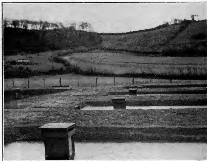
CONTROLLING SLUICES IN PONDS.
