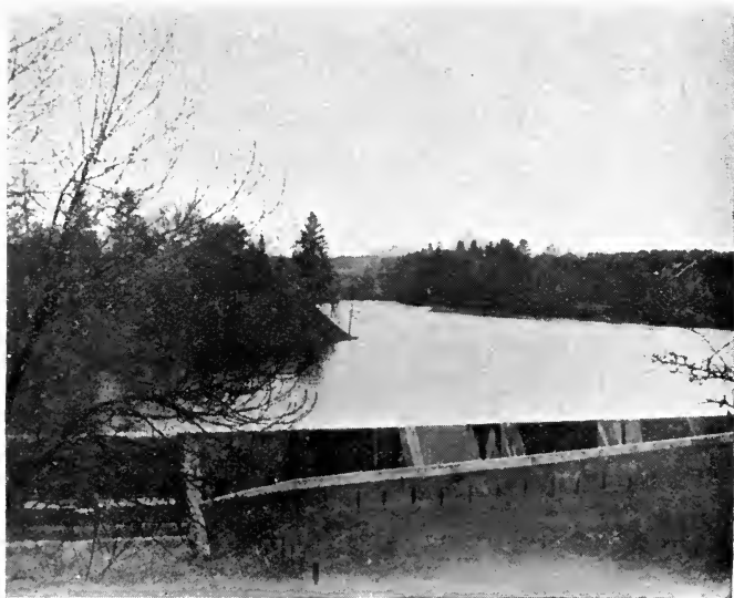
THE LAKE, FISH-PASS, AND DAM AT BATTLEBY.
