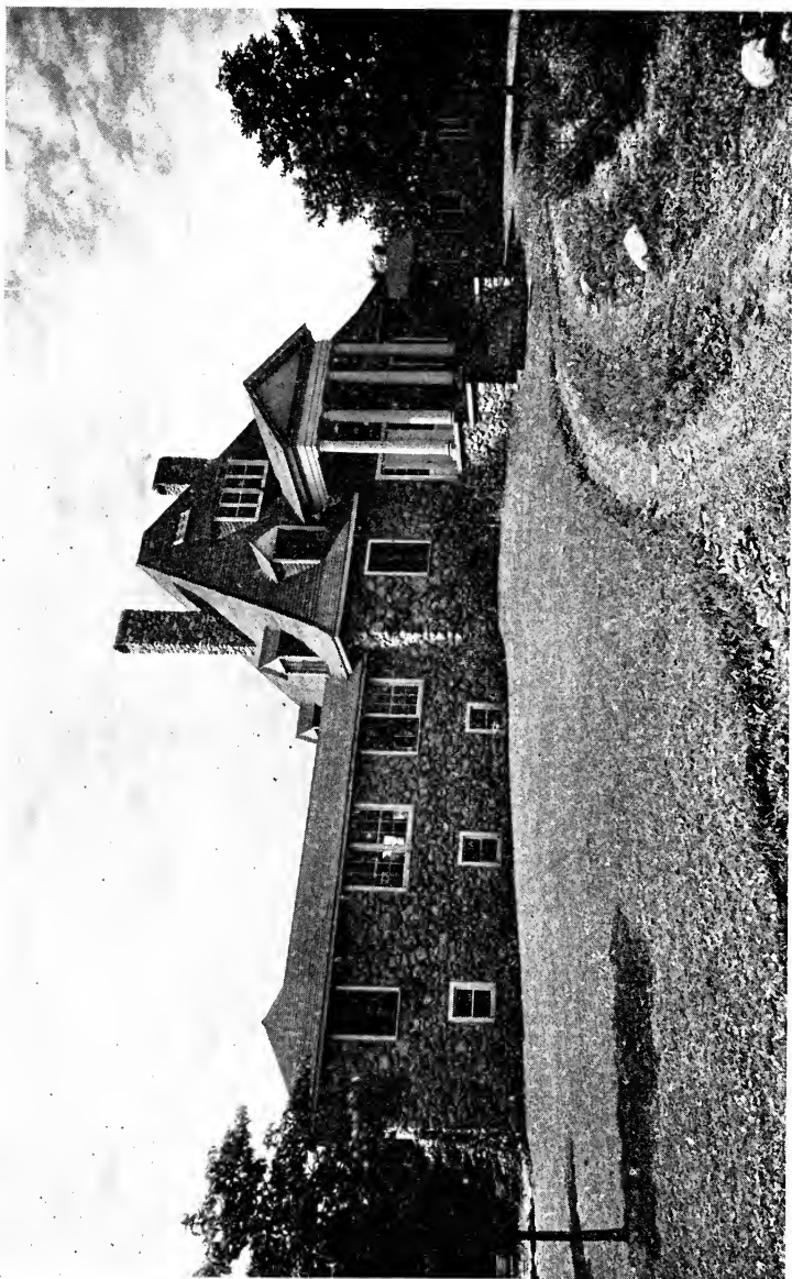
"Dogwoods," the Main House on the Homestead. One of the Wings Contains the Workshop, the Other the Loom-room. Designed and Built by Amateur Labor. Even the Wiring, Plumbing, and Steam-fitting Were Done by What Can at Best Be Described as Semi-skilled Labor. The Stonework in All the Houses on "Dogwoods" Was Put in by Amateurs, Using a Modification of the Flagg Method of Wall-building.
