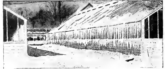
Here is what happens in the winter to the southern eave of Mr. S. Goddard's wooden plate house at Framingham, Mass.
