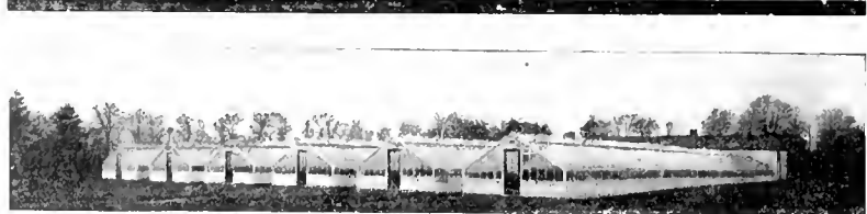
Six Iron Frame Orchid Houses erected for Julius Roehrs & Sons. These houses are equipped with our Galvanized Iron Frame, Tile Bottom Benches.
