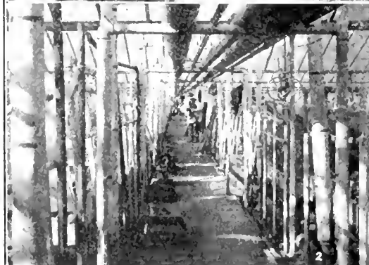
12. Showing how manure is handled from cars. The fork seen at left on trolley is operated from hoisting engine in small house at right. Three men do unloading with this outfit where twelve were required before. Plant A.
