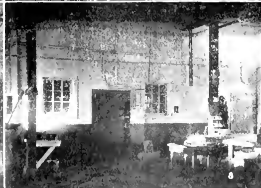
13. Cement manure tank, of Pochtmann's, Plant A, for making liquid manure. Man is keeping screens in receiving vat free.
