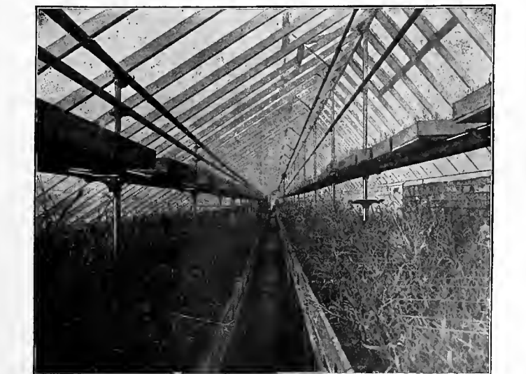
Greenhouse Showing Economy Bracket in Place
