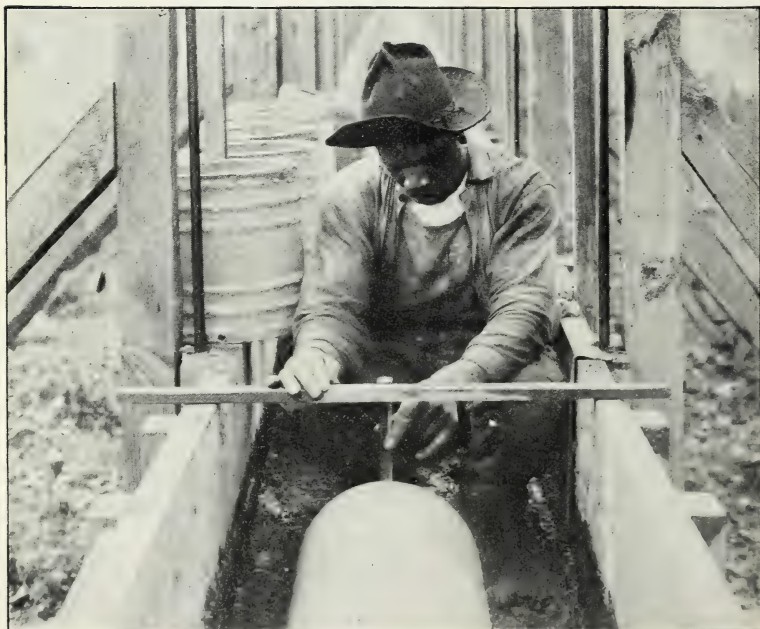
FIG. 2.—LAYING 10-INCH CONCRETE TILE IN THE FLUME.
