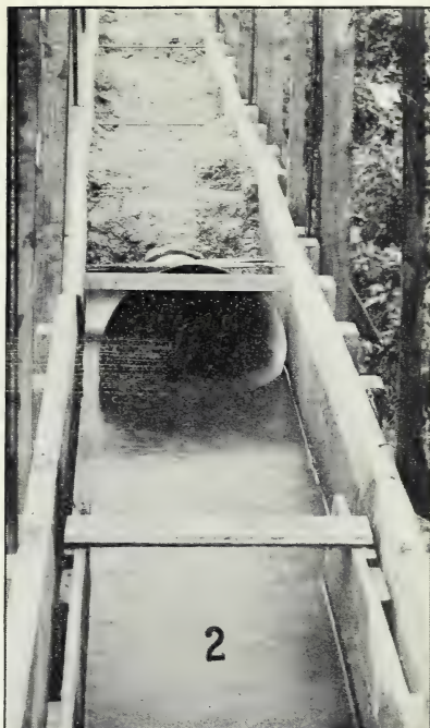
FIG. 2.—CONICAL ENTRANCE USED TO INCREASE ENTRANCE VELOCITY INTO TILE.
