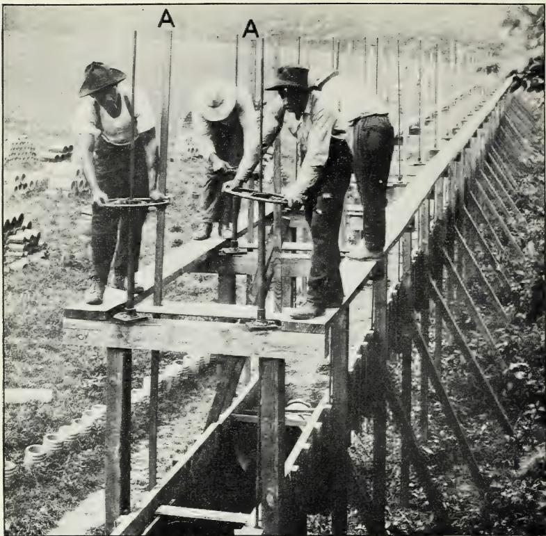
FIG. 1.—CHANGING THE GRADE OF THE FLUME.
