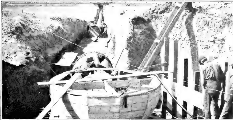
FIG. 1.—SIPHON UNDER UNION PACIFIC RAILROAD, ROCK CREEK CONSERVATION CO., WYOMING.
