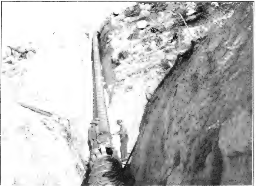
FIG. 2.—PIPE FOR BUTTE, MONT., MUNICIPAL SUPPLY. (No. 32.) SPRINGING IN A BUCKLE JOINT.
