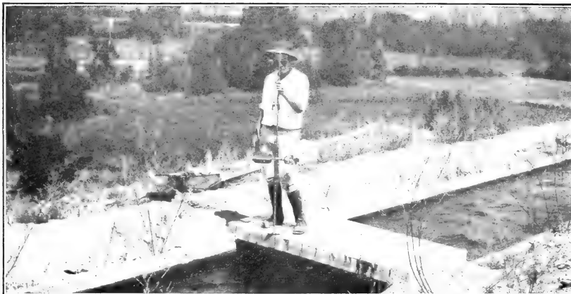
FIG. 3.—CURRENT METER STATION BELOW OUTLET TO PIPE No. 42.
