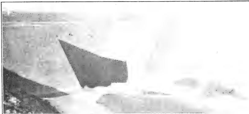
FIG. 3.—WINTER FLOW IS RETARDED BY SLUSH ICE. Note rings for grating removed to prevent ice accumulation.
