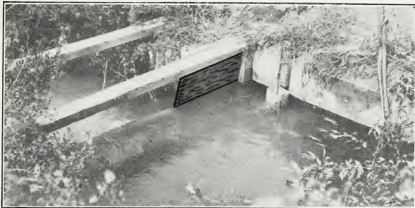
FIG. 1.—TYPICAL CIPOLLETTI WEIR, WITH HOOK GAUGE IN STILLING BOX. Note brush screen in foreground to reduce velocity of approach.
