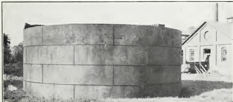
FIG. 3.—TANK OF BUTLER (PA.) WATER CO. USED IN MEASURING DISCHARGE OF PIPE NO. 29.
