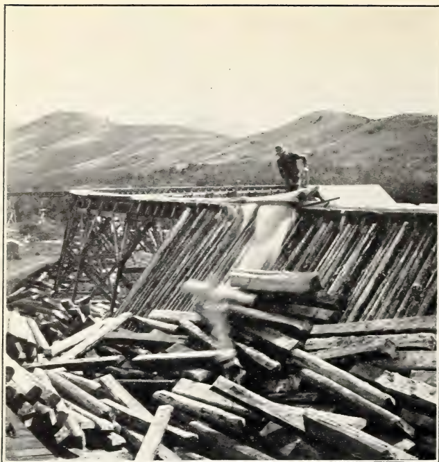
FIG. 1.—A "SNUB" IN OPERATION, THROWING CROSSTIES OUT OF FLUME AT RAILROAD LANDING BY PRESSURE OF WATER.
