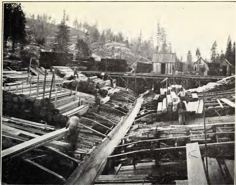
FIG. 1.—BRAILING AND ACCOURTRING LUMBER AT THE UPPER END OF A FLUME. Note the sloping "ways" on which the brails are slid into the flume after being clamped.
