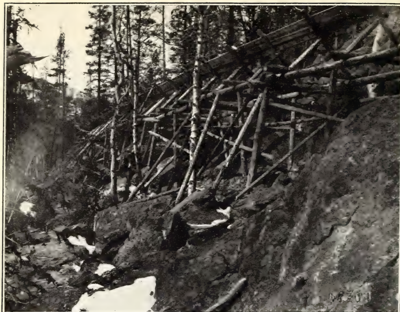
FIG. 1.—A FLUME IN THE CONSTRUCTION OF WHICH SMALL ROUND TIMBER WAS USED FOR EVERYTHING EXCEPT THE "BOX."
