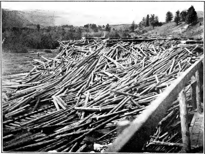
FIG. 2.—A "MINING STULL" DUMP AT THE LOWER END OF A FLUME WHERE THE STULLS ARE RUN DIRECTLY OUT OF THE "VENT" ENDS.
