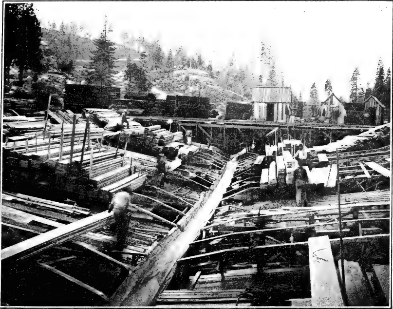
FIG. 1.—BRAILING AND ACCOURTING LUMBER AT THE UPPER END OF A FLUME. Note the sloping "ways" on which the brails are slid into the flume after being clamped.
