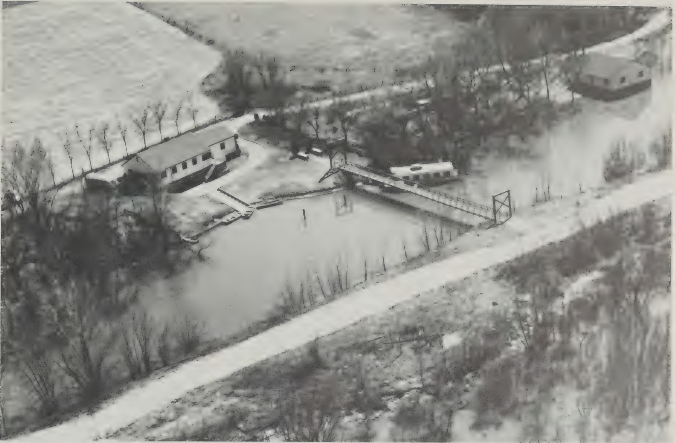
During the depression years of the 1930s, the federal government established work programs that made possible a variety of construction projects. The Survey made use of that opportunity to construct a building to house the Havana Station. The frame structure was completed in 1940, a mile or so from the site on Quiver Lake where Forbes had established the station in 1894.
