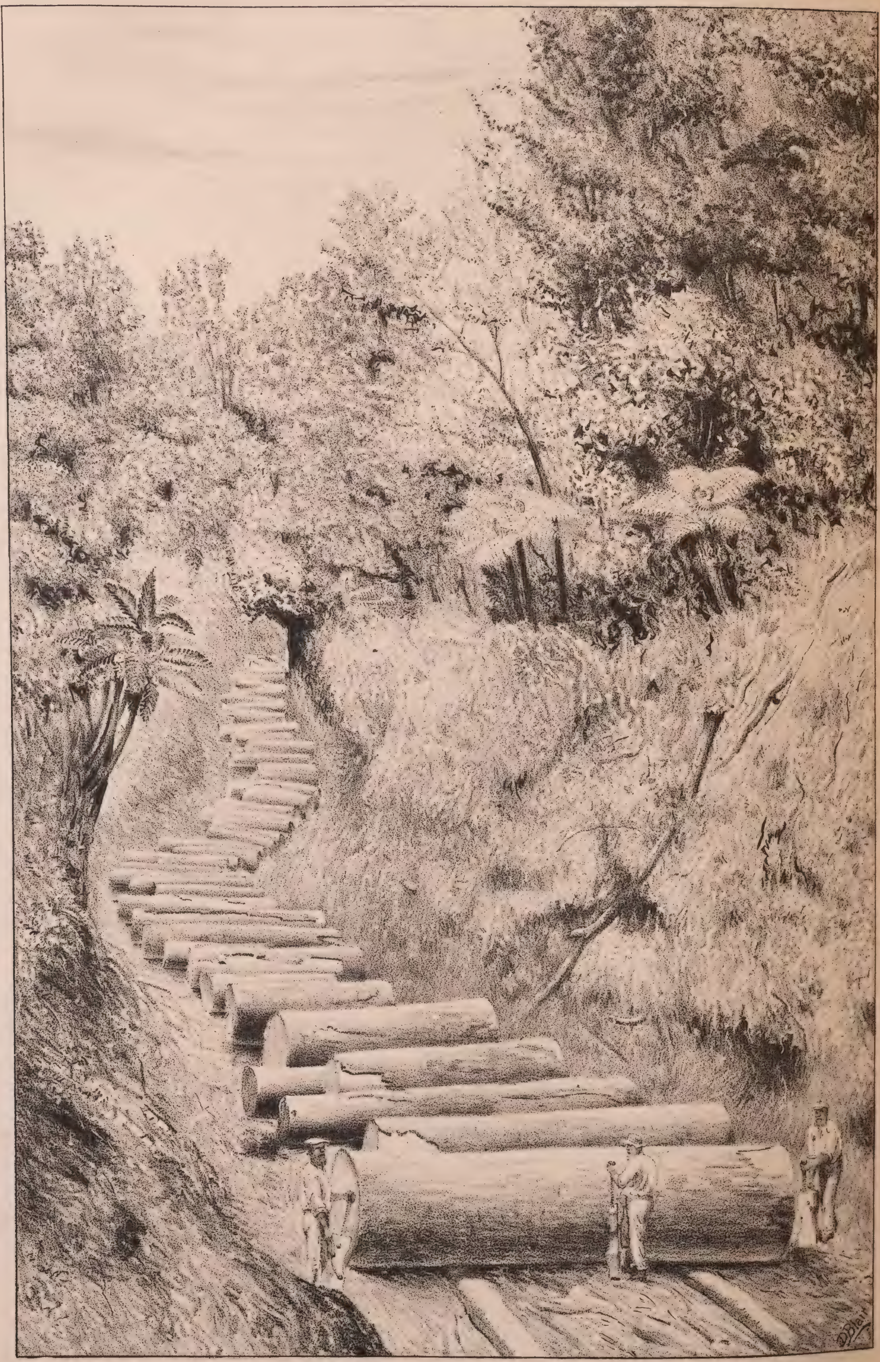
Kauri Logs on a Rolling Road. From a photograph by Foy Brothers.
