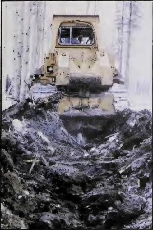
Ripper Plow Scarification
