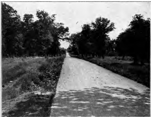
CONCRETE ROAD LEADING TO PRESERVE.
