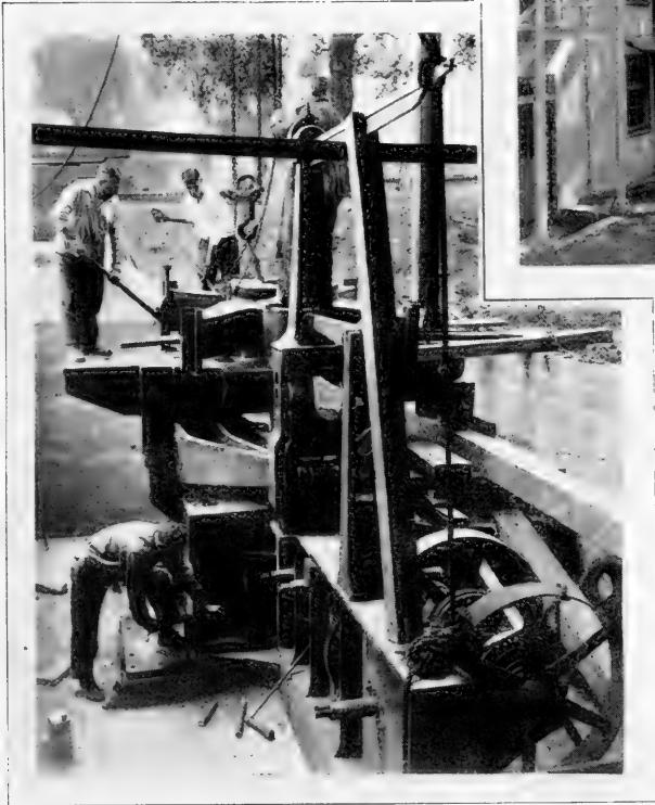
ERECTION OF THE MILLION POUND TIMBER TESTING MACHINE (1920)
