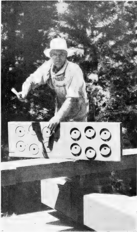
Modern metal connectors act as dowels or keys in the construction of strong timber joints.
