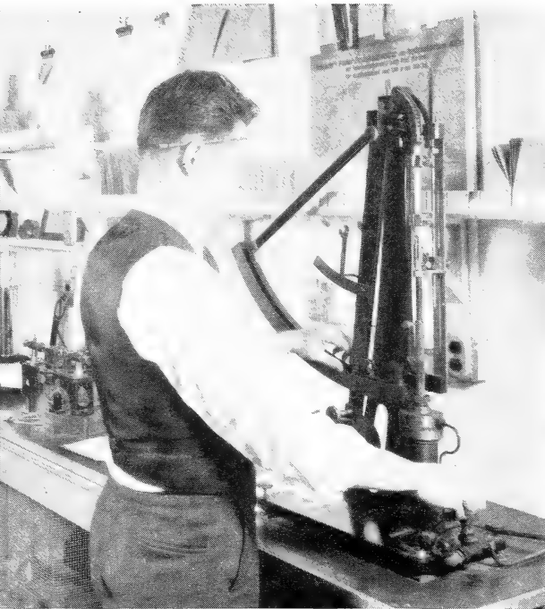
The tensile test—one of many tests used in evaluating paper quality.
