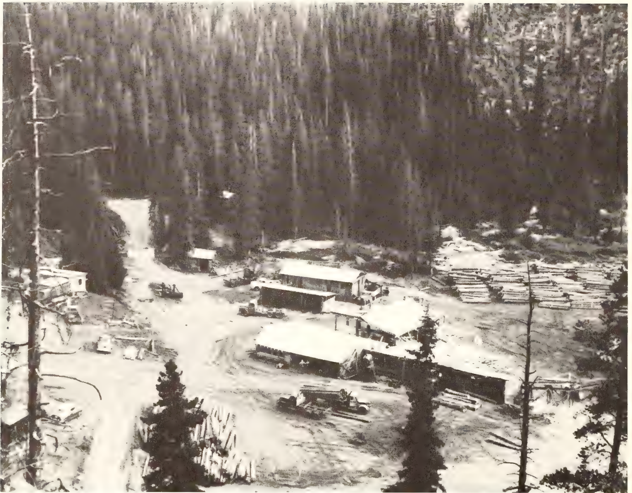
This small sawmill on the Colorado State Forest in Jackson County operates on small lodgepole pine and Engelmann spruce saw logs. It is representative of the numerous small mills in northern Colorado.
