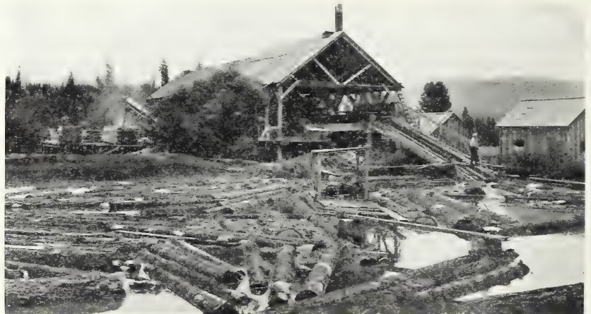
FIGURE 28.—Circular sawmill in western Washington having a capacity of approximately 30,000 board feet per 8-hour shift. The chief products of small mills are railroad ties, planking, timbers, common boards, and dimension. Usually such mills are located in the woods near their log supply
