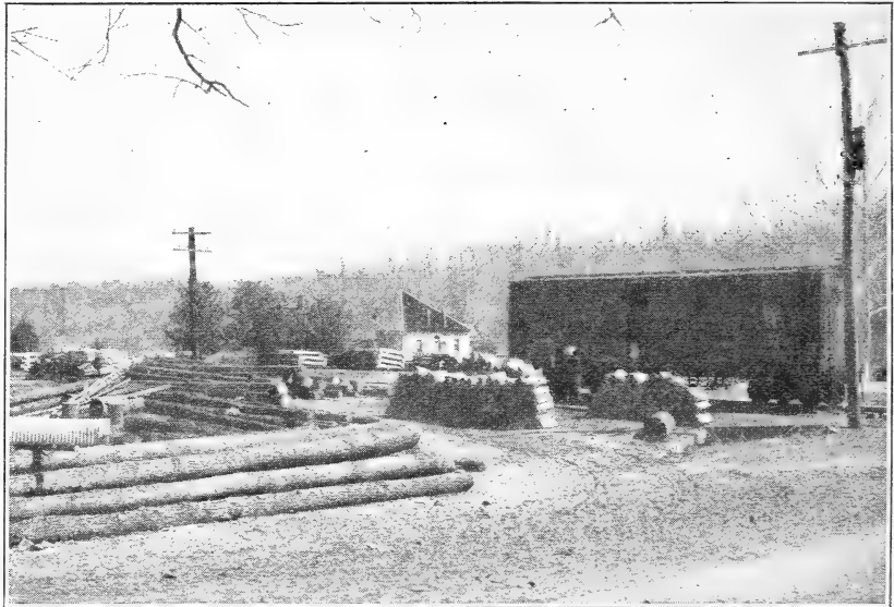
FIG. 11.—Oak spoke blocks, piling, and crossties ready for shipment.
