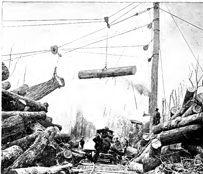
(Tree Rigged Cableway Skidder Pulling and Loading Logs)
