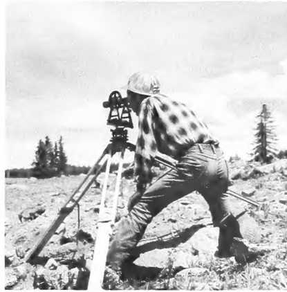
Engineers surveying for a new road in Grand Mesa National Forest, Colorado. The layout of this road was done from aerial photographs using the latest photogrammetric techniques.
