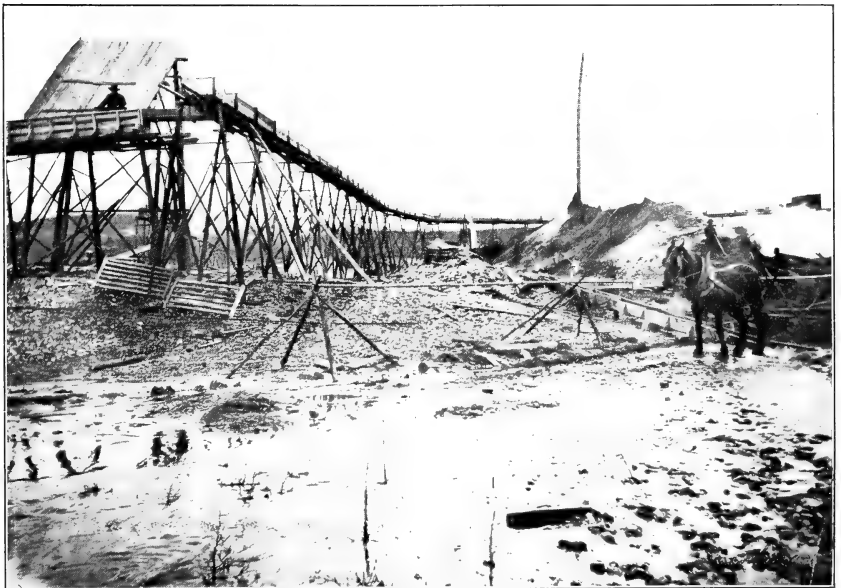
FIG. 2.—TYPICAL FLUME AND SLUICE BOXES USED IN PLACER MINING FOR GOLD IN THE FAIRBANKS DISTRICT. MUCH LUMBER AND MANY POLES ARE REQUIRED FOR THESE PURPOSES.
