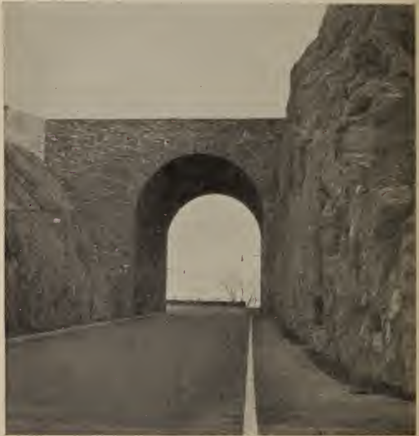
The great arch, cut in the schist rock of the ridge on which Fort Tryon Park stands, to provide an automobile entrance from Riverside Drive. The rock from this cut was used for walls and buildings in the Park.
