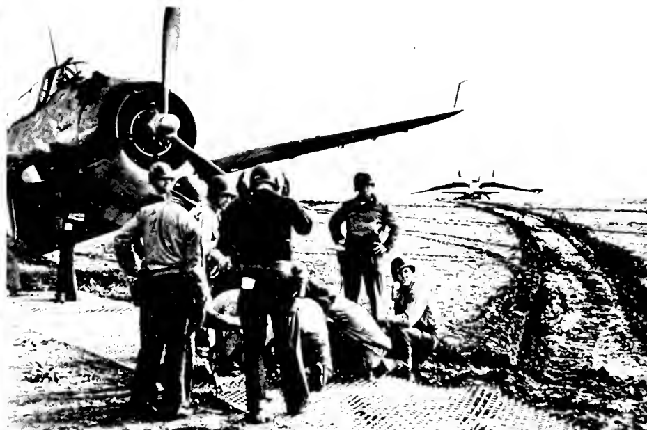
Seabees build landing fields on muddy wastes
