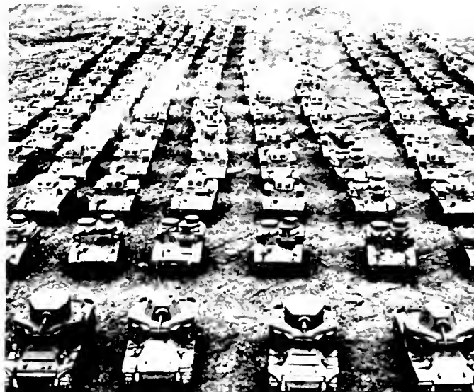
Tanks, tanks and more tanks
