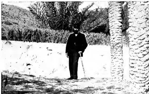
FIG. 7. — Typical sand wall topped with date-palm branches in use at Tozeur, southern Tunisia.
