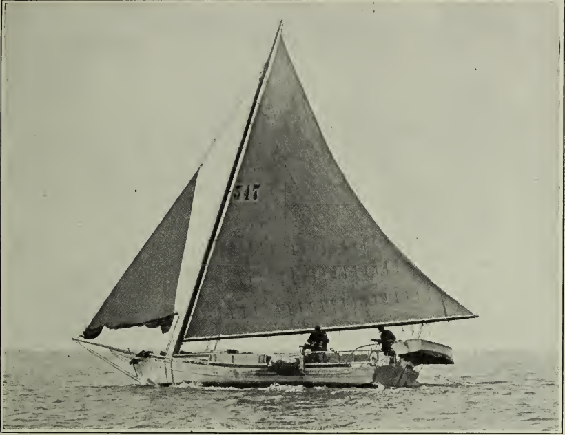
FIG. 1.—SMALL SLOOP OR "SKIP-JACK" USED IN DREDGING OYSTERS IN CHESAPEAKE BAY.
