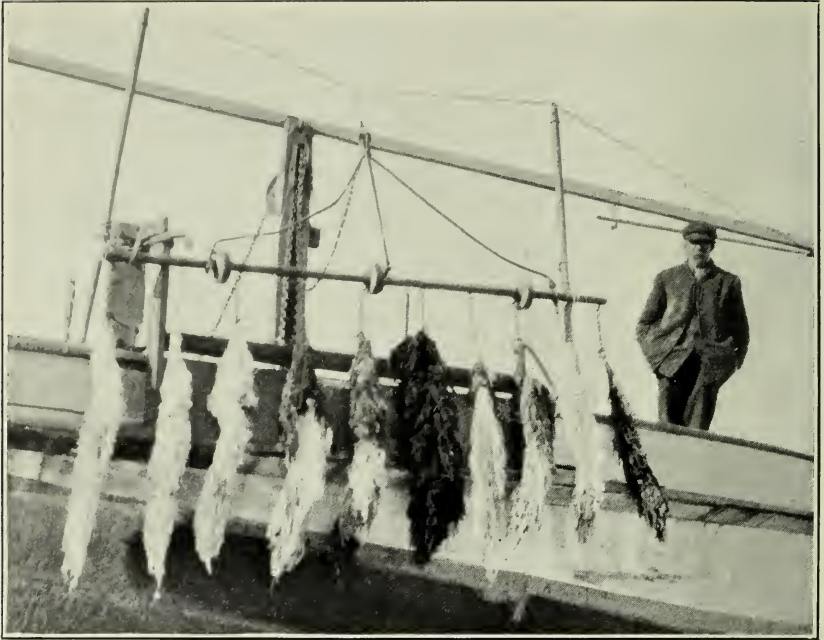
FIG. 1.—USUAL STYLE OF "STAR MOP" USED FOR EXTERMINATING STARFISH IN LONG ISLAND SOUND.
