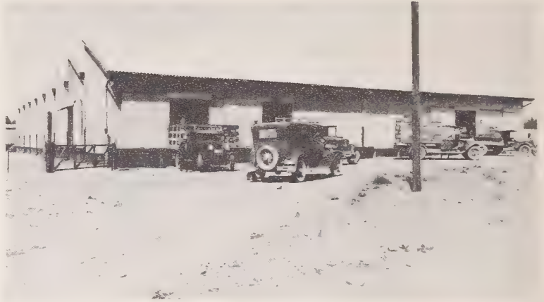
FIGURE 31.—Exterior of one of five similar sheds operated by the Argentine Fruit Distributors in the Río Negro Valley. The construction is simple, inexpensive, efficient, and easy to enlarge. (Courtesy of Great Southern Railway.)
