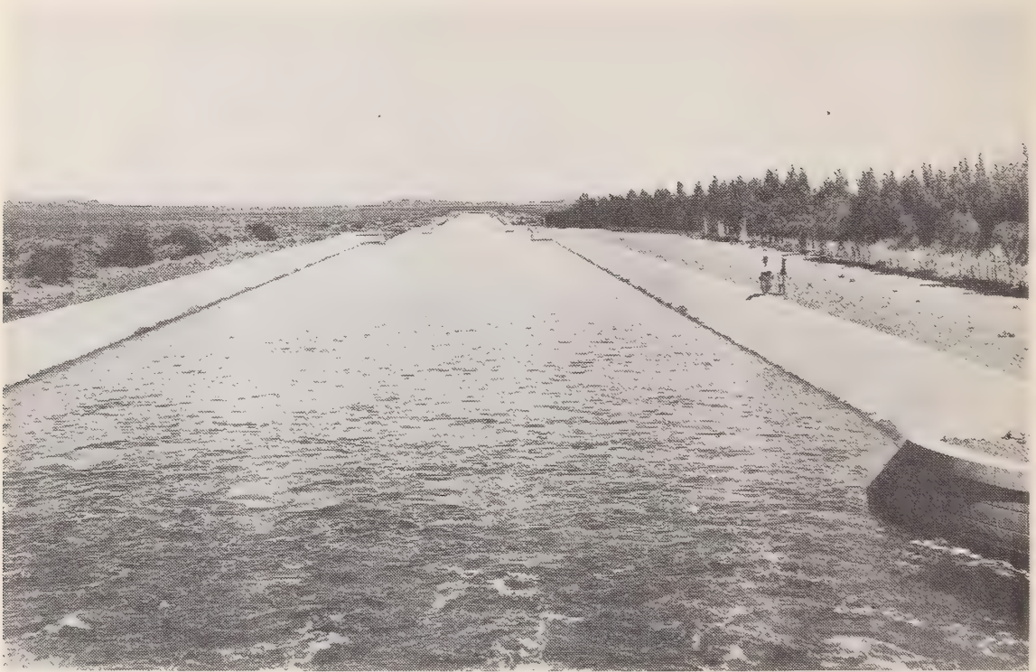
FIGURE 7.—Main canal diverting water from the Neuquén River at Contralmirante Cordero. Note windbreak at right. (Courtesy of Great Southern Railway.)
