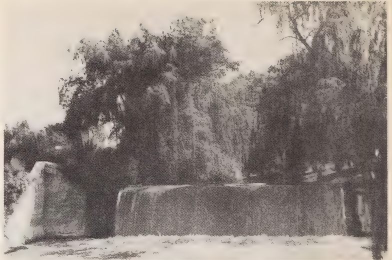
FIGURE 11.—One of the many small dams used to divert water from natural streams in Mendoza.
