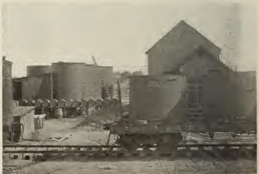
THE LATIMER CIDER AND VINEGAR PLANT AT GRAND JUNCTION
