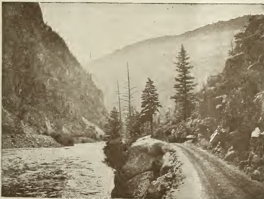
SAMPLE OF ROAD CONSTRUCTION IN A PICTURESQUE COLORADO CANON
