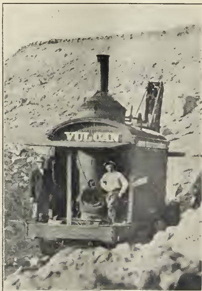
SIXTY HORSEPOWER VULCAN STEAM DITCHER ON MAIN CANAL
