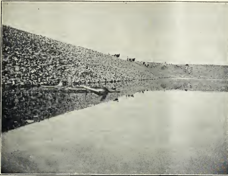
VIEW OF A SECTION OF STORAGE RESERVOIR ON COTTONWOOD CREEK
