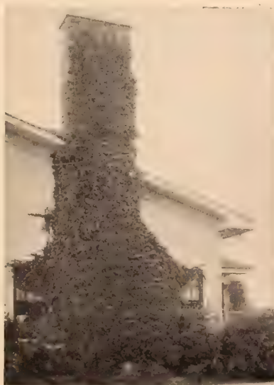
Ivy Covered Chimney
