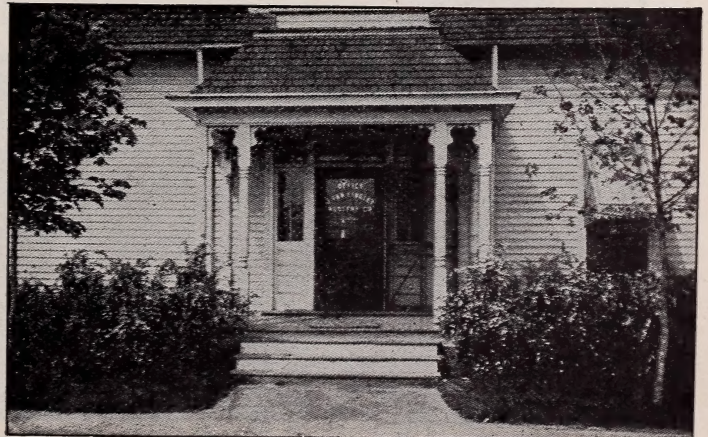
This shows the same place after planting
