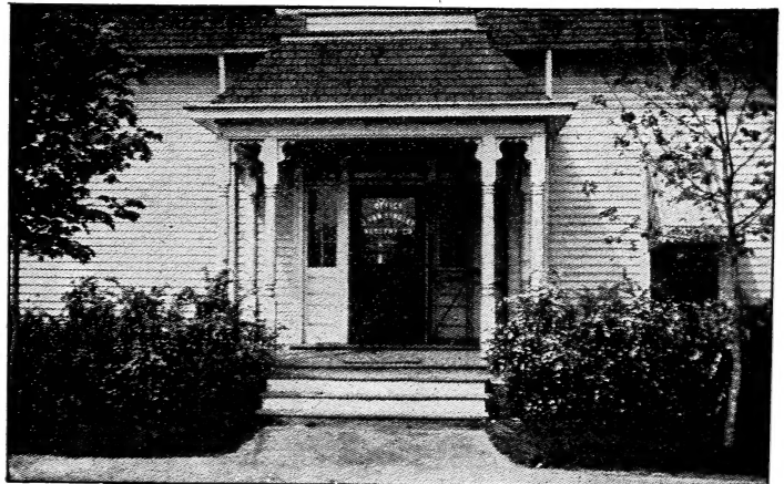
This shows the same place after planting
