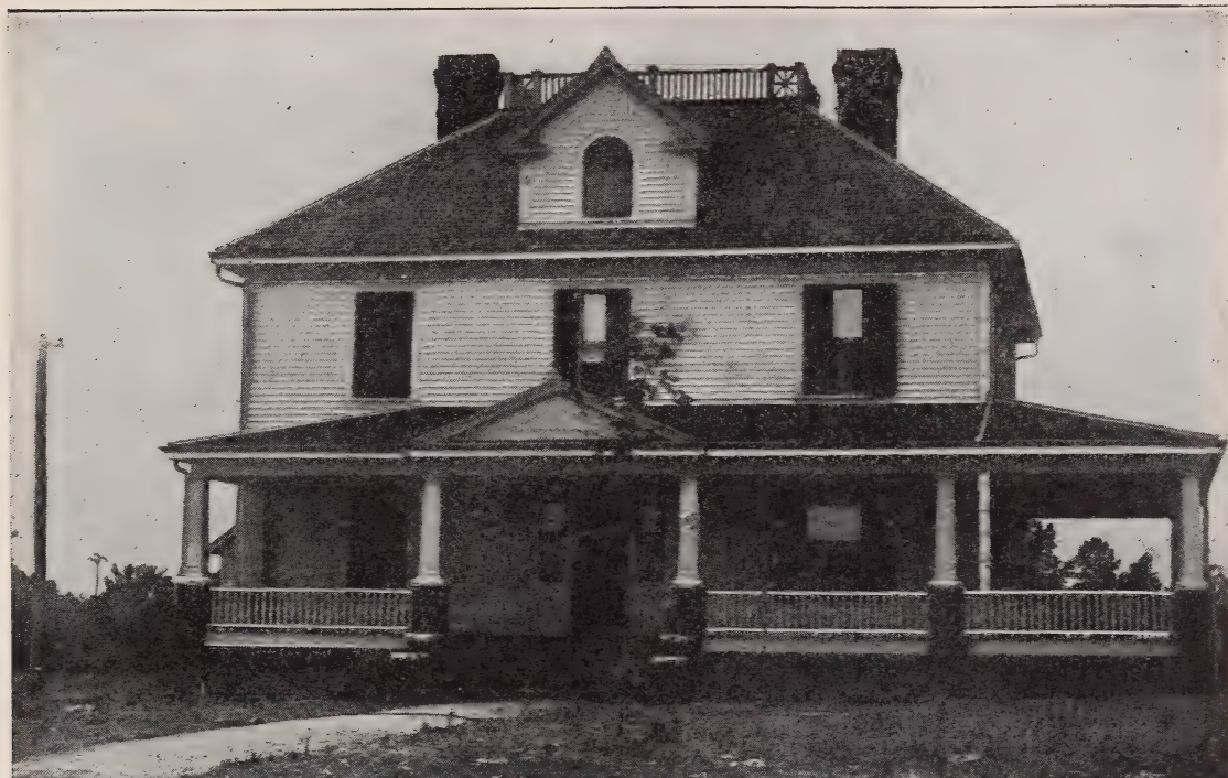
A suburban residence near Pomona, N. C. The photograph was taken before any planting had been done around the foundation walls or about the lawn
