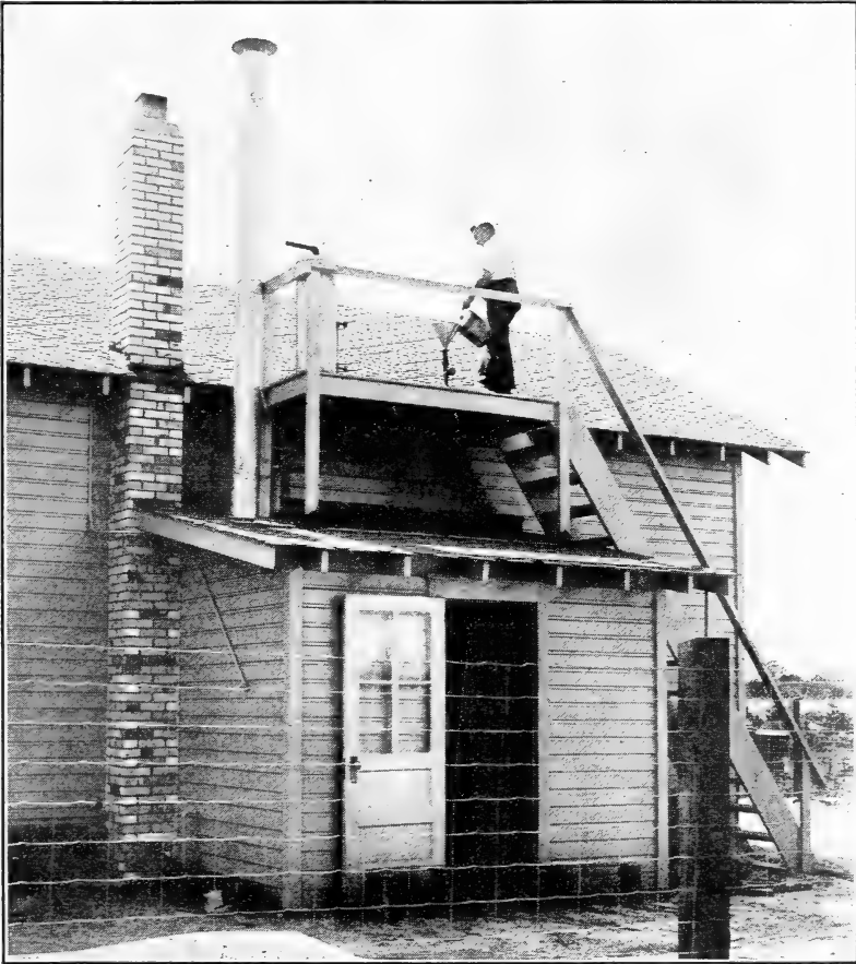
FIGURE 12.—Pouring carbon disulphide into the evaporating pan at the fumigating plant at Hamonton, N. J.
