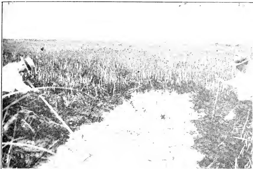
The first blast of dynamite blows out a pirogue trail of sufficient width and depth. The sticks for future explosions are set in the burned grass area at the end of the water hole.
