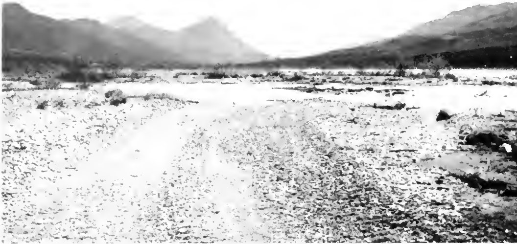
Figure 73. Compacted surface gravels in an access road leading to the Dietrich River-Downstream site.
