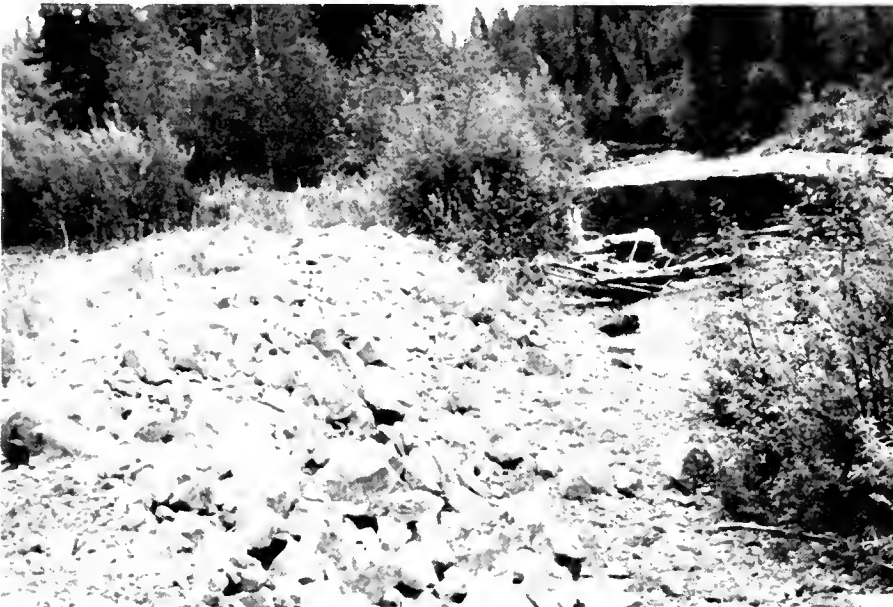
Figure 84. Armored bank protecting the West Fork Tolovana River pit from a channel diversion into the mined site.
