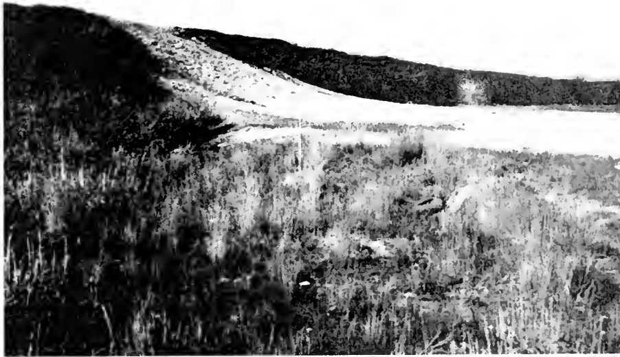
Figure 82. Gravel fill ramp used to protect the incised bank at the Sagavanirktok River study site.
