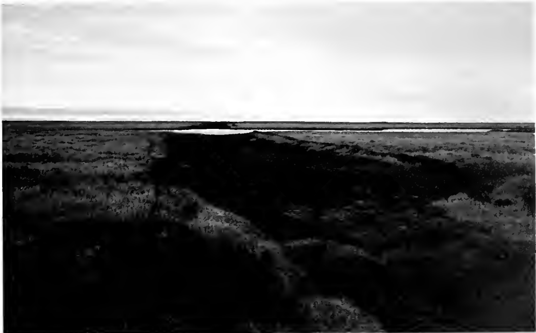
Figure 92. Thermal erosion near Ugnuravik River resulting from compaction and destruction of the vegetative mat overlying ice-rich permafrost soils.
