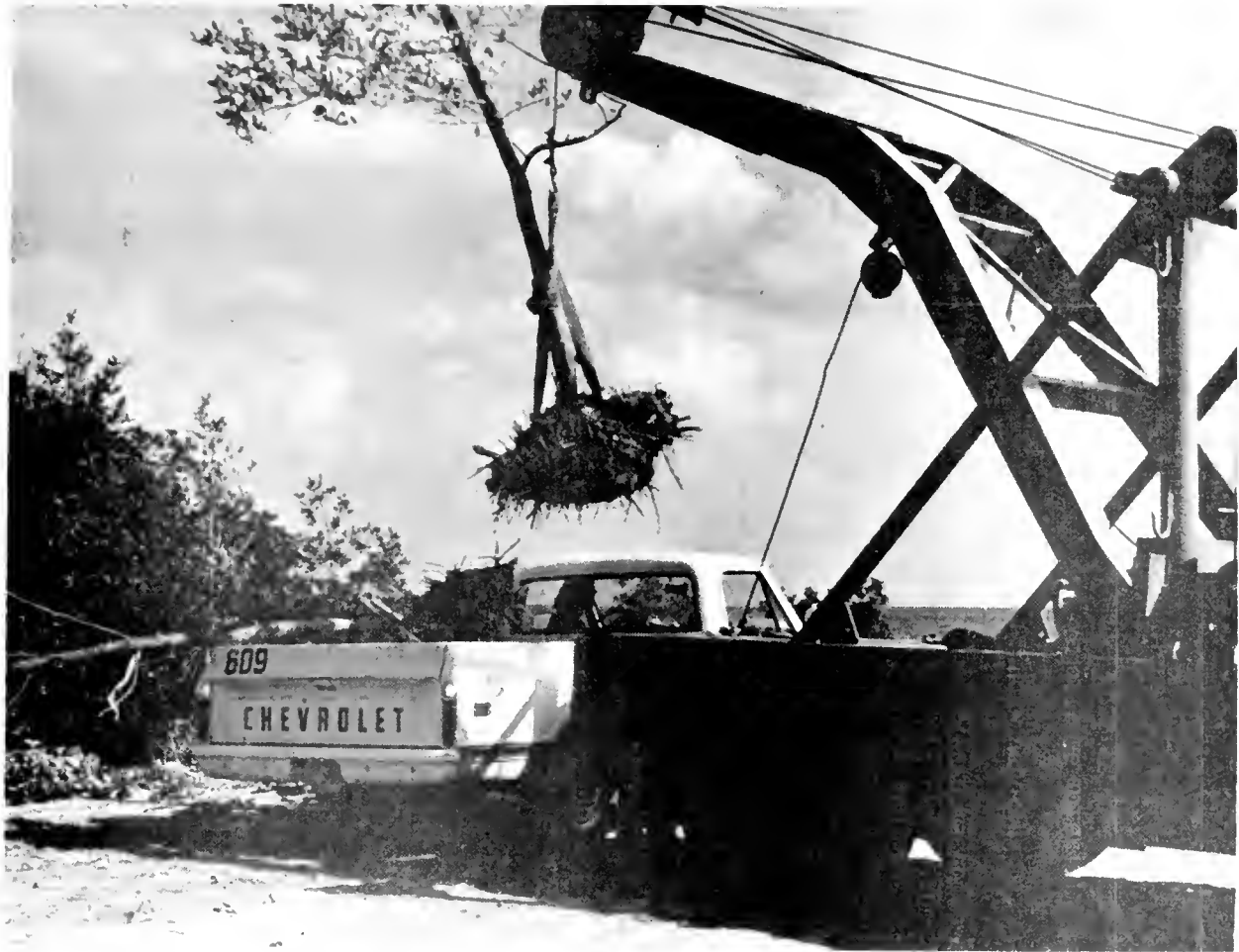
Figure 20. Black mangrove being moved for transplantation by use of a tree crane.
