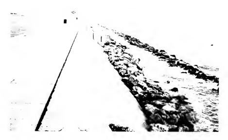
Figure 4. Western part of massive seawall on Galveston Island. Note lack of sand beach seaward of the seawall.
