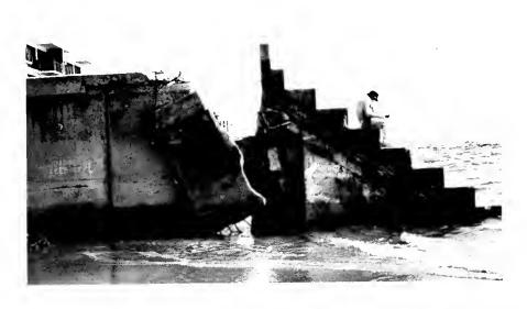
Figure 6. Seawall on North Padre Island damaged during Hurricane Allen.
