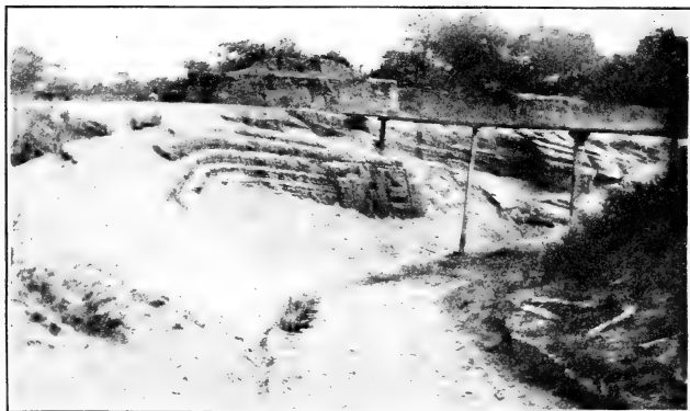
SAND-PIT SHOWING CAUSE OF EXTREME DRYNESS IN SOME PARTS OF TOWN.
