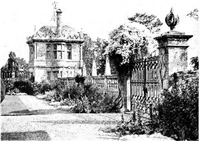
PAVILION IN THE FORECOURT AT MONTACUTE, SOMERSETSHIRE.
