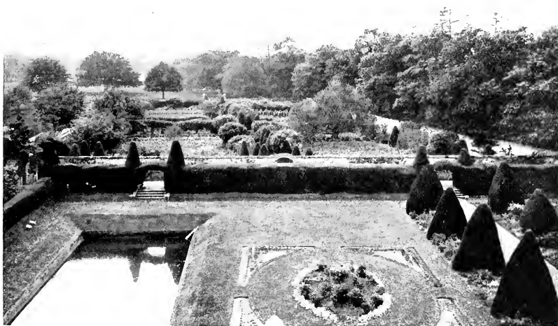
STEW-POND AT BRICKWALL, SUSSEX.
