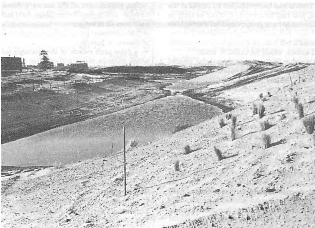
A view of part of the parkland under construction.
