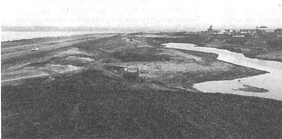
Another view of the work under construction. Photograph by David Whitworth.
