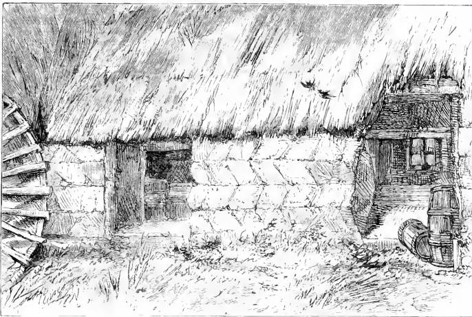
FIG. 49.—WOOD MILL: SHOWING CONSTRUCTION OF THE WALLS. (SEE P. 339.)
