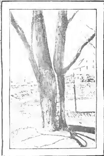
Excavated and casted to 17". Note how concrete has filled in the cavity, section on section for sealing and preventing decay. Note also view of Pilgrim on the background.
