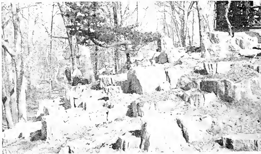
Rockgarden construction at "Lindenhurst." Pocket building on a steep grade.
