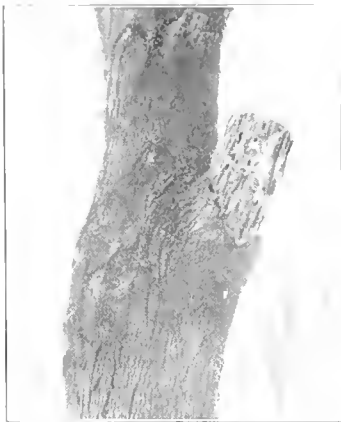
IMPROPER PRUNING, leaving the exposed stub open to the attacks of disease fungi, is sure to result in decay which eats progressively into the trunk. Davey experience and scientific training have taught the Davey Tree Surgeons how to make this operation a permanent success in every case. Daveyite, the best wound dressing ever produced, is used to protect the wounds.
