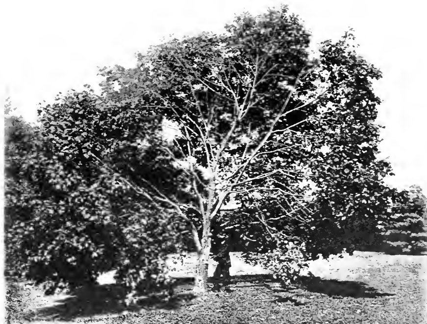
T: an untrained eye the crotch of this neglected forked maple tree appeared to be perfectly safe for, as will be seen, very little decay is noticeable. In this tree as in all V shape crotch trees, it is necessary to support the crotch against high winds and side strains, by the use of cables and bracing. These braces are most important; and should not be inserted in any slip-shod way, otherwise more damage than good will be the result. A man skilled in the work will insert these cables and braces in quick order, and at the same time, insure the natural sway of the limbs, and the proper flow of sap and the healing over of any wounds. The picture shown plainly denotes a beautiful specimen tree with one side entirely ruined. Arthur M. Horn.
